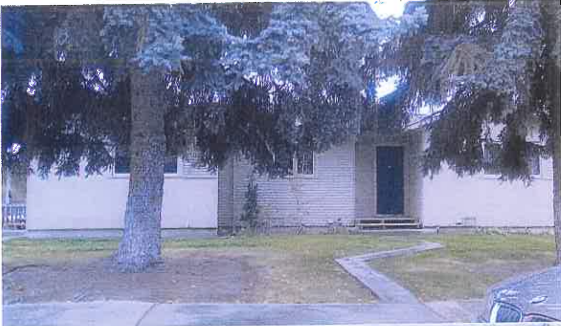
GLENWOOD AVE DUPLEX
